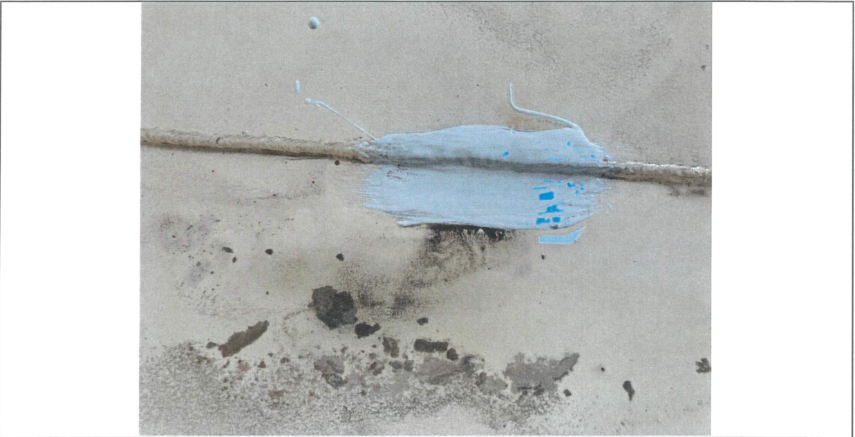
AFTER Completed coating repair
