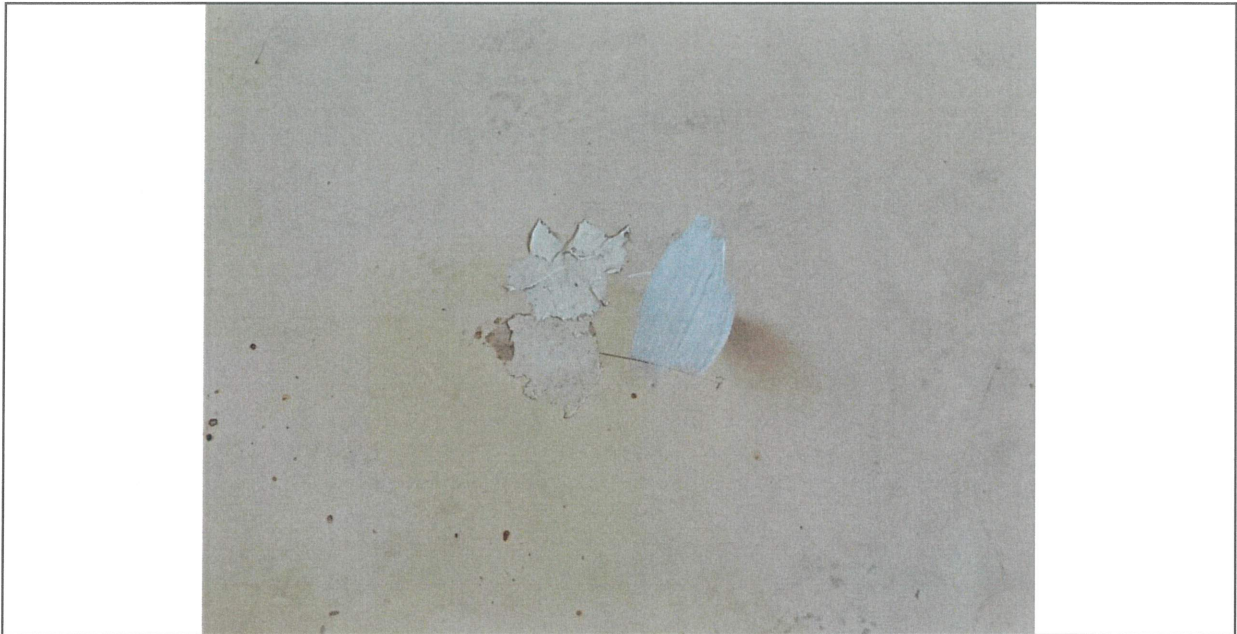
AFTER Completed coating repair
