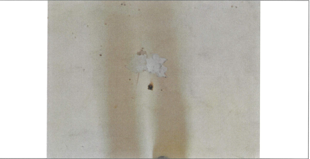
AFTER Completed Wash
