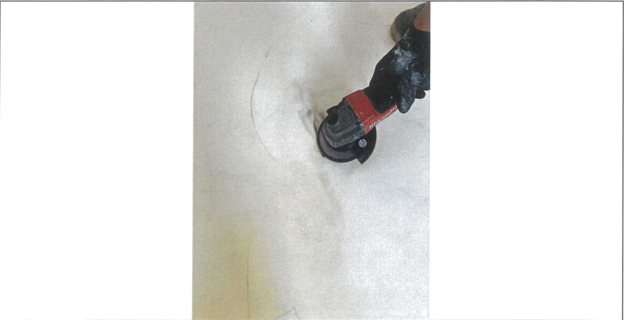
AFTER Surface preparation on repair areas
