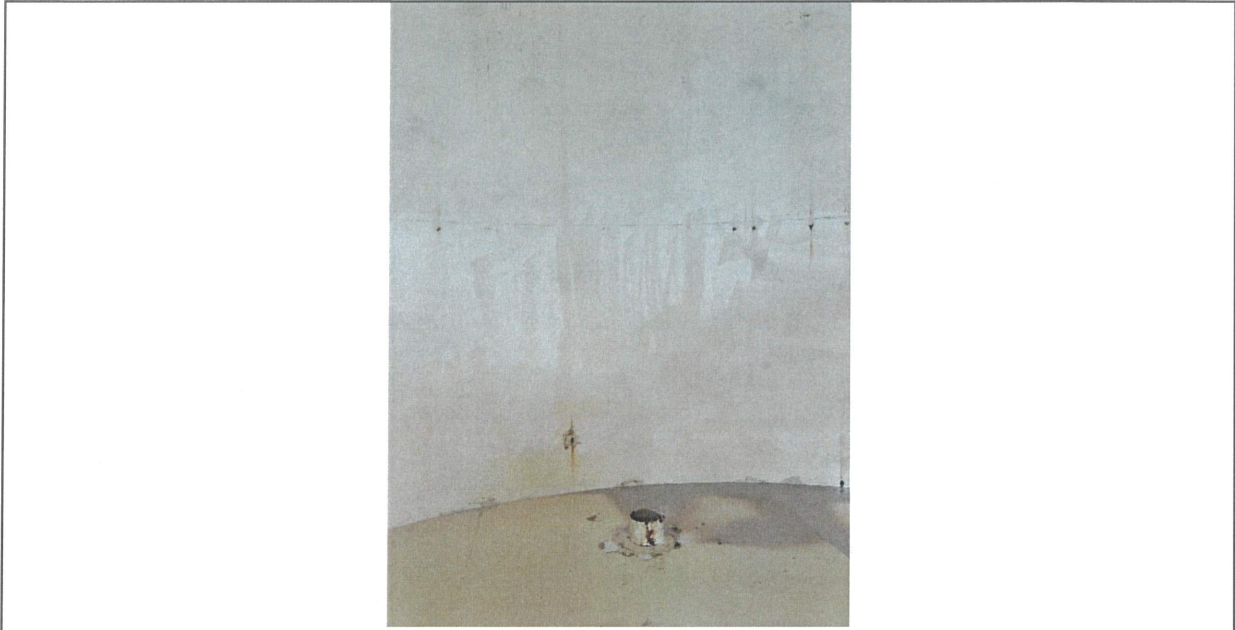
AFTER Completed Wash
