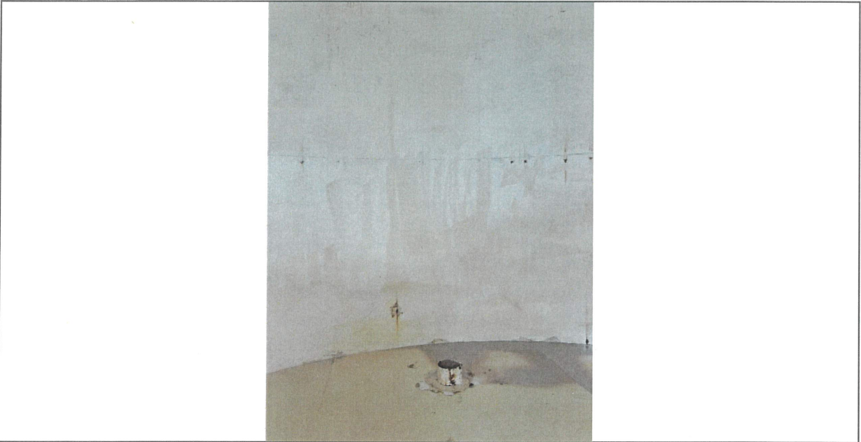
AFTER Completed Wash
